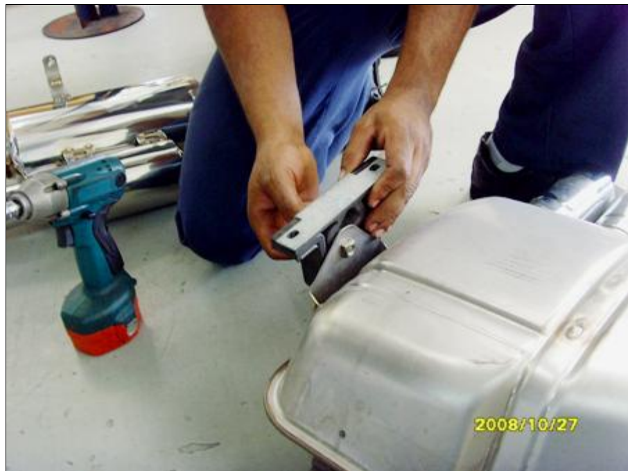
Disconnect the right exhaust hanger from the factory rear muffler
